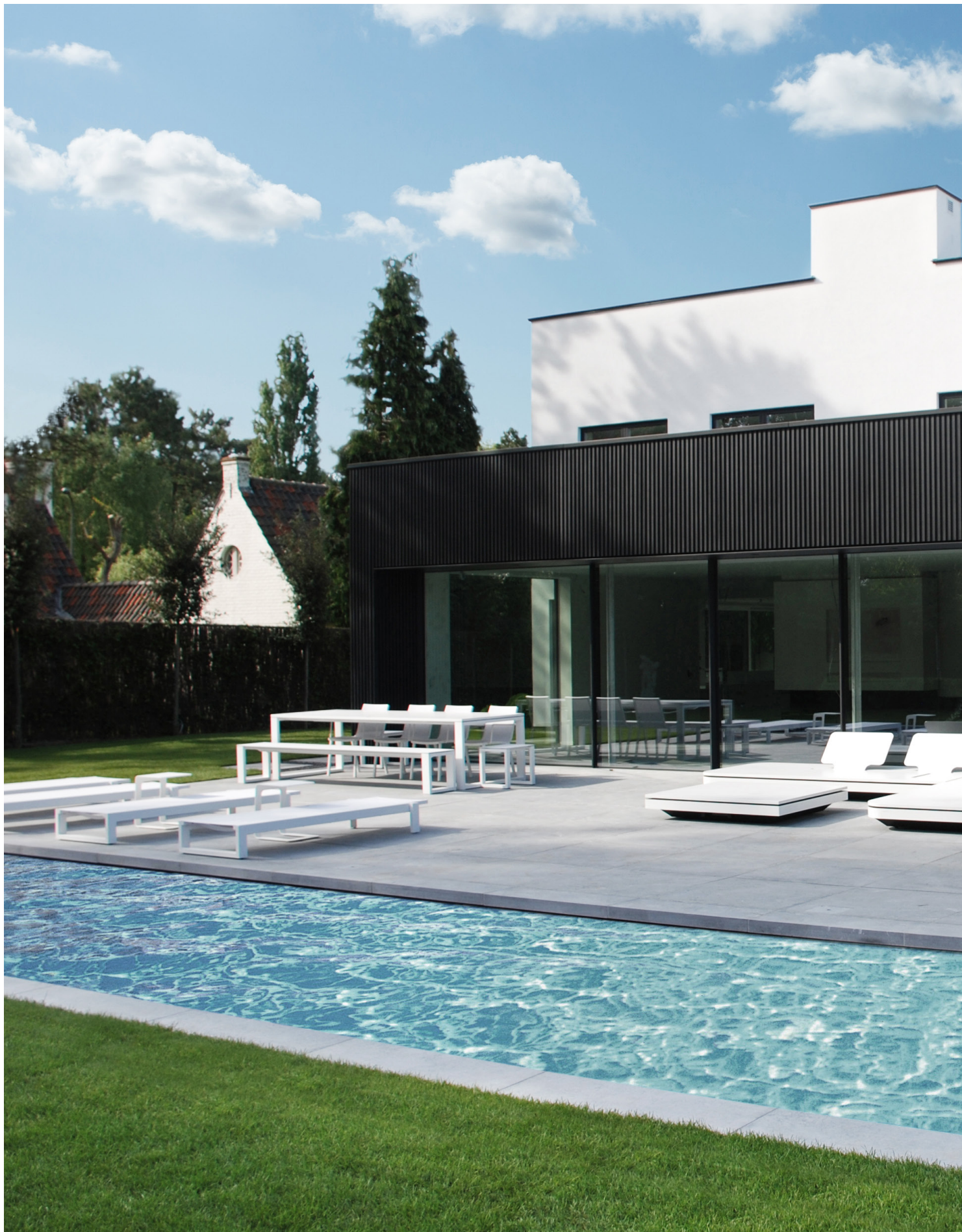
©Dubois Houtskeletbouw | Ainel A Serie | Architect: Arttec - Hans De keyser
